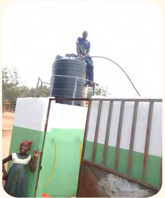
MAKING OF THE WATER TANK
